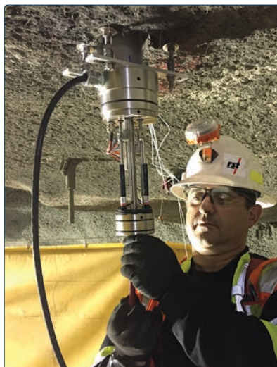
A Borehole Extensometer, with the Electrical Head cover removed, is being installed into the ceiling of an underground opening.
